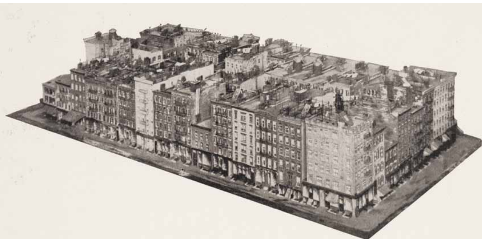
MODEL OF BLOCK ON LOWER EAST SIDE From the Tenement House Exhibition of 1900
